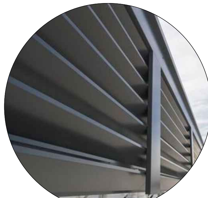
2 MECHANICAL EQUIPMENT ROOFTOP LOUVERED ALUMINUM SCREENS
